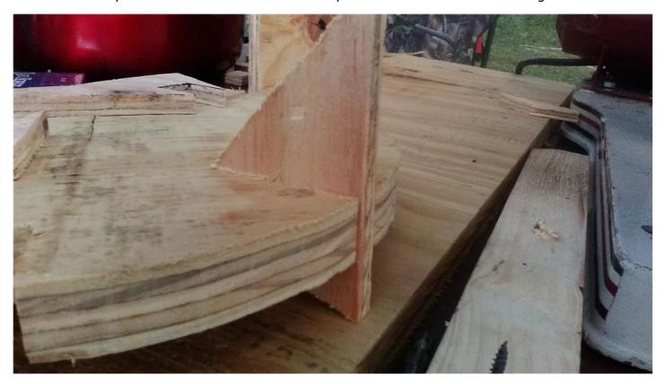
Glue in each brace and secure them till they dry. I use just a piece of rope or strapping. Basically whatever I have lying around. You can even do it with heavy twine. Just wrap around the outside to keep them from falling out. I usually use liquid nails for projects like this because of it's gap-filling qualities.
